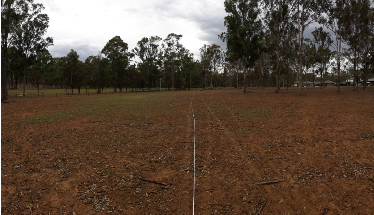
Photo 8 - Raked ground layer in the cleared areas after extensive dry period - centre of the western portion of the site looking towards the existing house and shed (November 2018)
